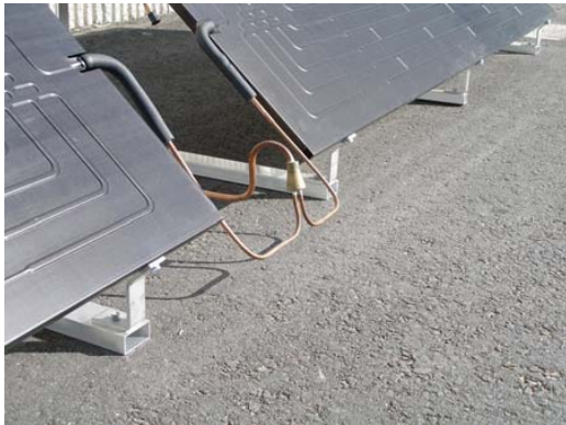
Fig. 18 Liquid distributor
